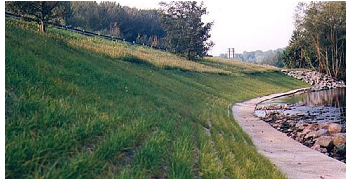
Photo source: River embankment, Gresford, Nr Wrexham https://www.externalworksindex.co.uk/entry/106743/Grass-Concrete/River-embankment-adjacent-to-the-A484-Gresford-Wales/
