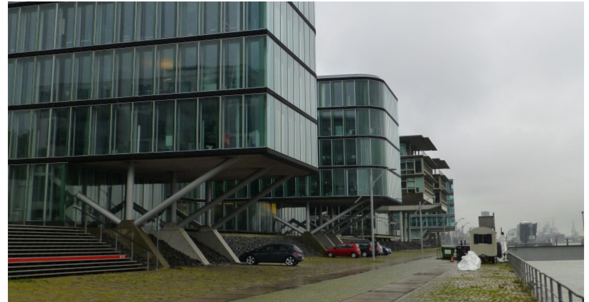
Photo source: Raised construction, Hafencity Hamburg © Mathieu Schouten https://www.urbangreenbluegrids.com/measures/measures-for-separate-buildings/raised-constructions/
