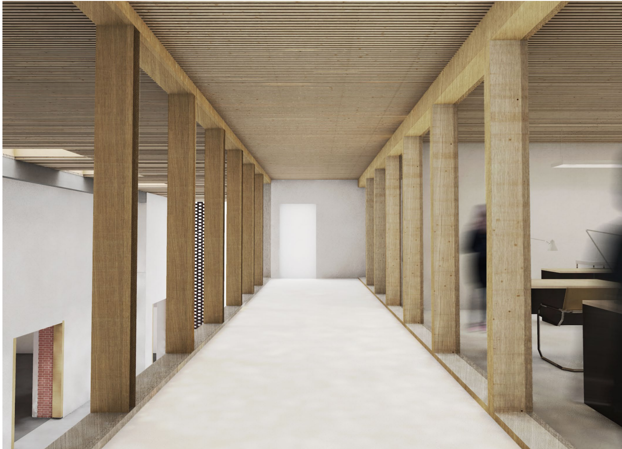
First Floor Corridor with Lignotrend ceiling
