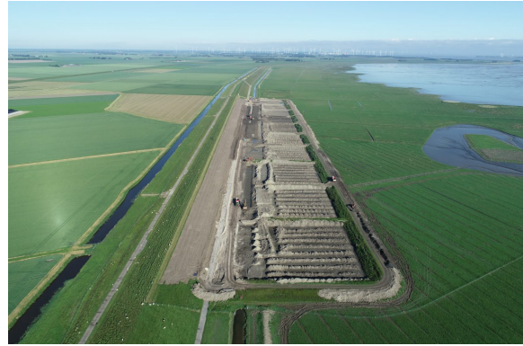
Figure 5.3: Aerial view of the construction of the Wide Green Dike (EcoShape, 2022)
