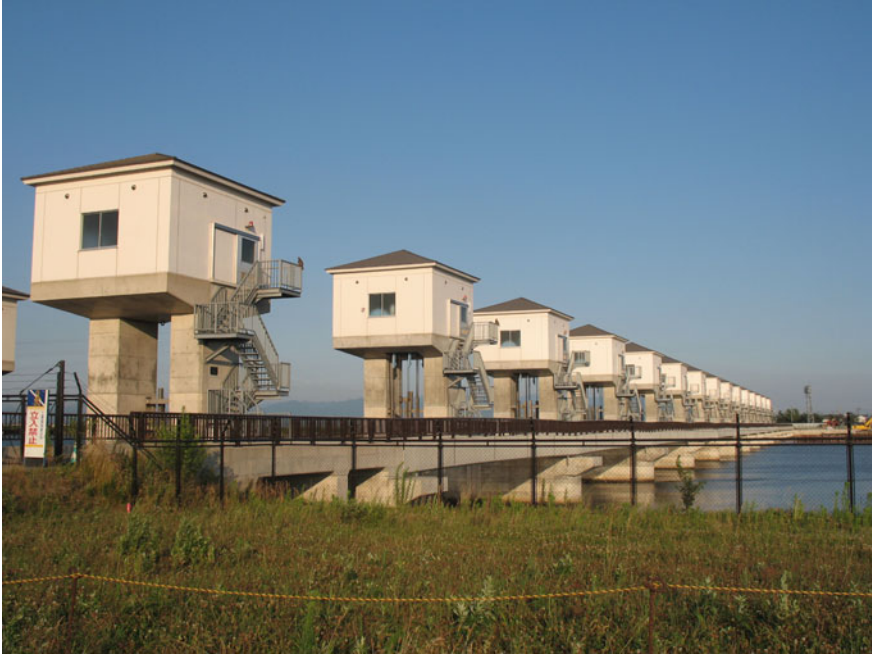
Fig. 13 Tide sluices of the Hachirogata lagoon. These tide sluices were built in 1961. This changed the remaining lake into a fresh water lake (Photo by Yasunori Kitao); released under a Creative Commons Attribution-Non Commercial-No Derivatives 4.0 International License
