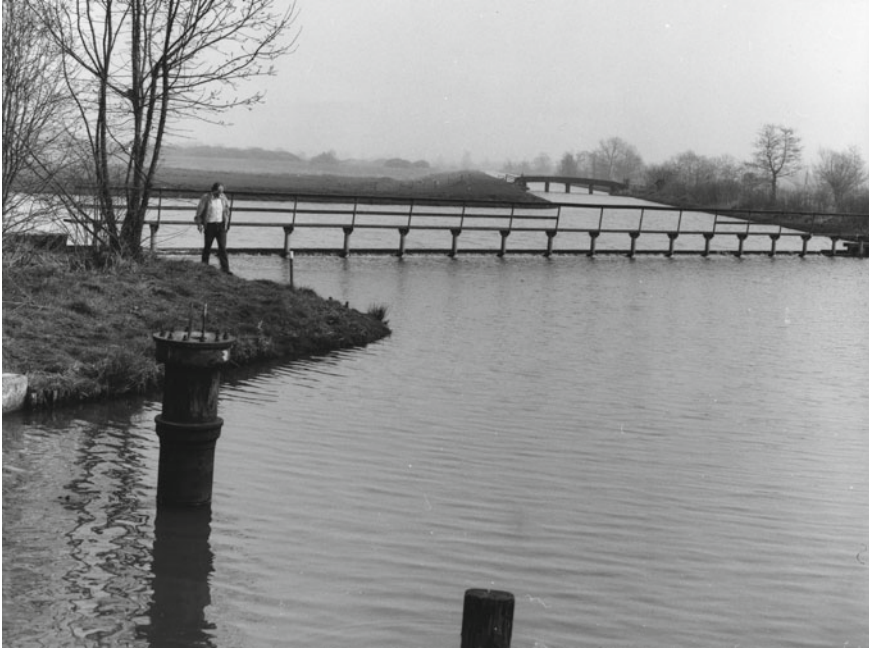
Fig. 14 Drinking water canal ( Waterleidingkanaal ) transporting seep water from Bethunepolder to the Loenderveenseplas for natural purification (ca. 1988). Source Het Utrechts Archief; released under a Creative Commons Attribution-NonCommercial-NoDerivatives 4.0 International License
