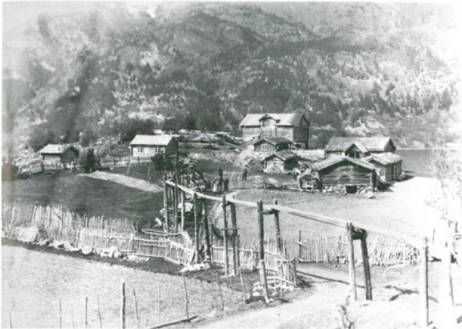
Fig. 12 Half-open wooden pipe to lead irrigation water at Søre Neset farm, Vågå, E-Norway ( Photograph Hans Joramo/De Sandvigske Samlinger Maihaugen); released under a Creative Commons Attribution-NonCommercial-NoDerivatives 4.0 International License
