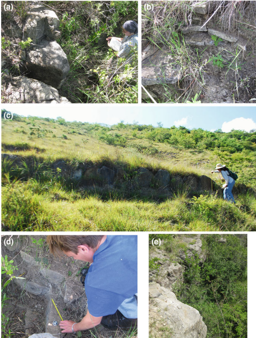
Fig. 5 a Canal and reservoir in stream north; b circular well in stream south; c wall that intersects stream north; d stepped well next to wall and inside stream north; e large reservoir at the end of streams north and south; released under a Creative Commons—Attribution-Noncommercial-NoDerivatives 4.0 International license
