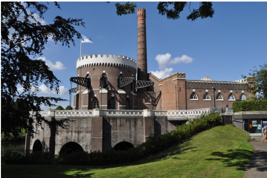
Fig. 3 HollandRoute Polderland Anchor Points Cruquius Steam Pumping House (Photograph: De Boer); released under a Creative Commons Attribution-NonCommercial-NoDerivatives 4.0 International License
