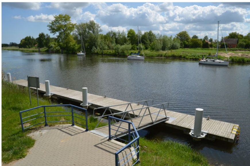
Fig. 14 Main water connection near Drewnica (Schönbaum, Photograph: De Boer); released under a Creative Commons Attribution-NonCommercial-NoDerivatives 4.0 International License
