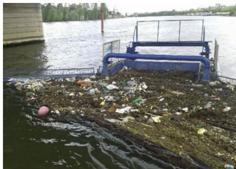
Figure 4: Surface litter collecting using an existing floating boom in the Seine (Gasperi et al., 2014).
