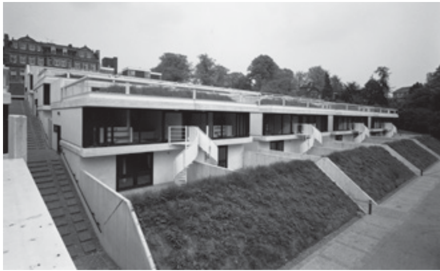
Exterieur, kort na oplevering Exterior, shortly after completion
