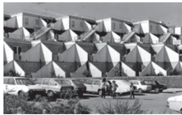
Hill Estate kort na oplevering Hill Estate shortly after completion
