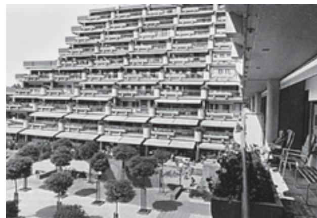
Woningbrede terrassen kort na oplevering Dwelling-wide terraces shortly after completion
