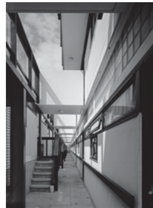
Fleet Road, laaggelegen steeg/ lower alley
