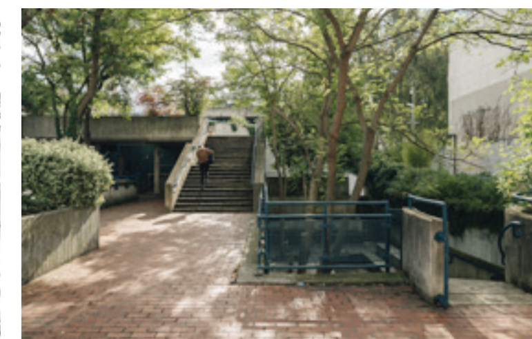
Alexandra Road, trap vanaf centraal plein/stairway leading from central square
