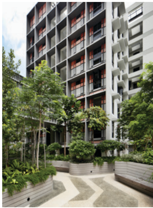
Entree woontoren vanuit daktuin Entrance residential tower from roof garden
