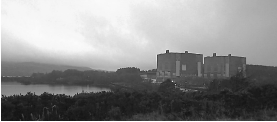
Fig. 5. View of Trawsfynydd 'cathedral like' reactor buildings from viewing platform next to site (Source: researcher's own, December 2017).
