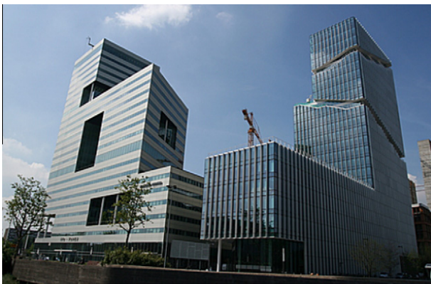
Fig. 8. Photograph of the real situation of case 2 (building on the right).
