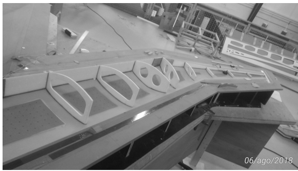
Figure 2.10: Manufacturing. Assembly of the structure on-going.
