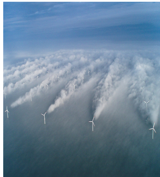
Figure 3.4: Wind Turbine Wake Effect at Horns Rev 2 (source: Vattenfall, 2017)
