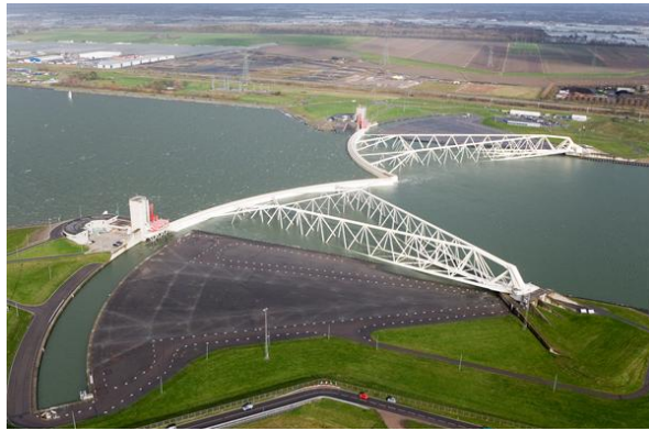
Figure 4.3: Example of a flood barrier: the Maeslantkering [76].
