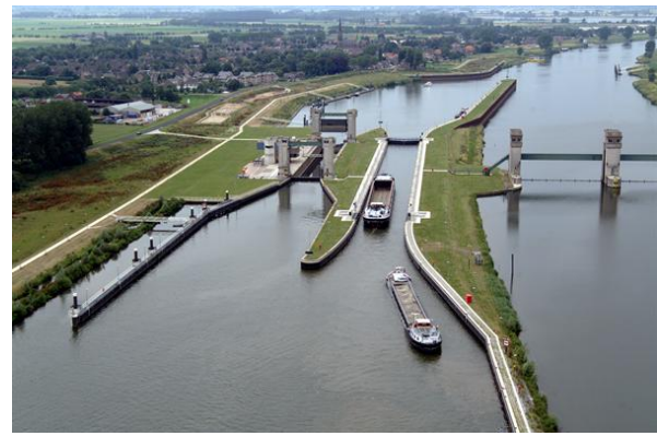
Figure 4.5: Lock at Lith (2 chambers) with a weir to the right [76].
