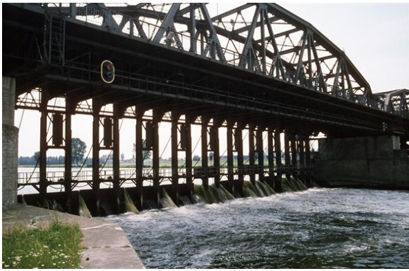
Figure 4.2: Example of a weir: the weir at Grave [76].
