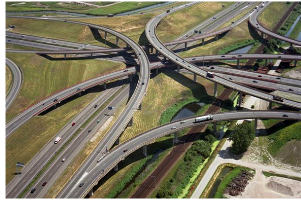
Figure 4.8: Road intersection Prins Clausplein, exchange of vehicles is possible between all directions [76].
