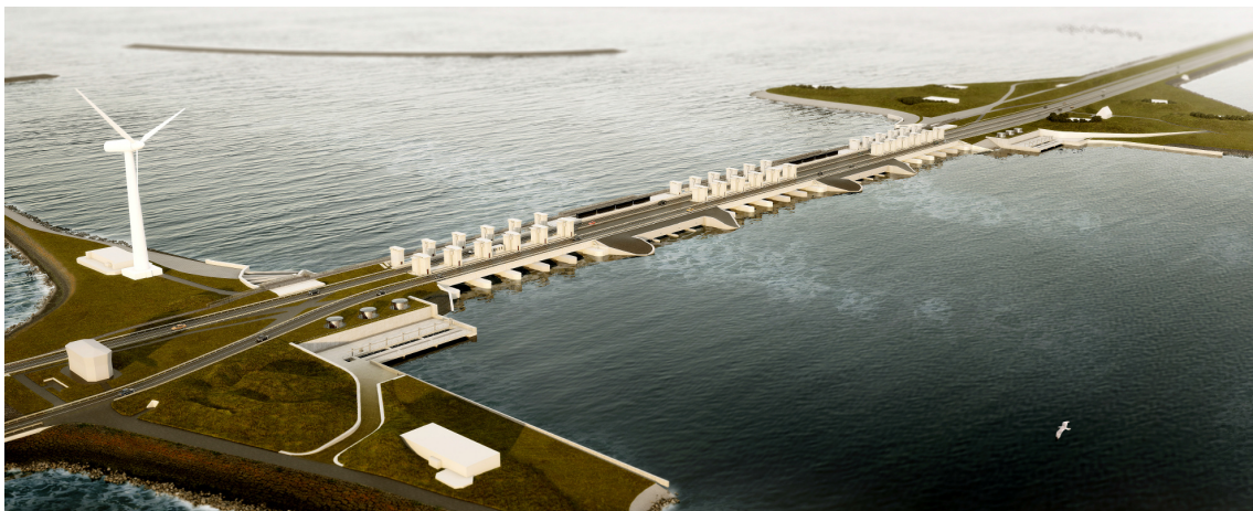
Figure 1.1: Animation of the renewed discharge sluices of the Afsluitdijk near Den Oever
