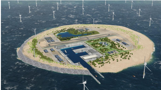
(a) Offshore artificial rock revetment energy island, adopted from reve (2024)
