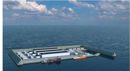
(b) Offshore artificial caisson energy island, adopted from Danish Energy Agency (2022)
