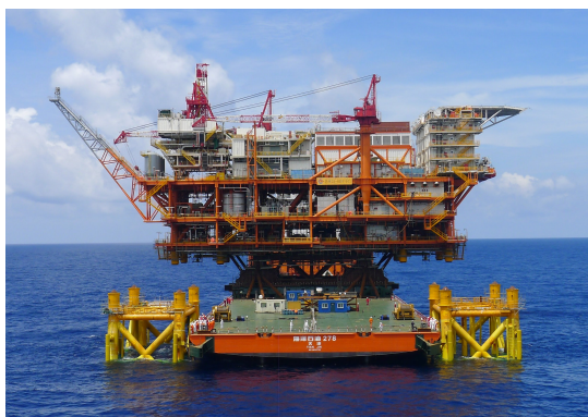
(a) Float-over installation of topside
