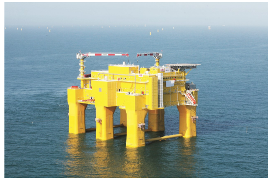
(b) Operation DolWin2 HVDC platform
