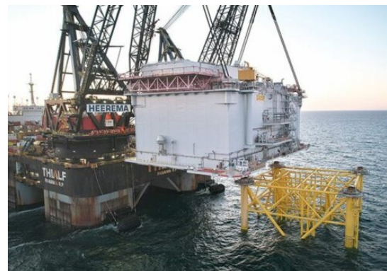
(b) Lift and set installation of topside
