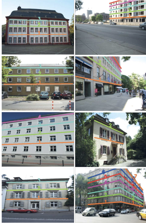
Figure 3.6.: The results of floor-level line detection with FloorLevel-Net, on more orthogonal view images (left) and perspective view images (right). Note how the floor-level line number corresponds to the number or count of the storey it is assigned to. In most cases, the highest floor-level line number corresponds to the floor count. Adapted from [Wu et al., 2021].
