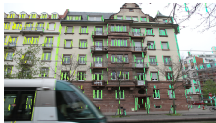
Figure 2.11.: Automatic rectification on singular façade images, that works by finding most prevalent horizontal and vertical line segments, which naturally reside in objects that are rectangular in the real world (e.g. windows and doors). As a result of the rectification, the lines in windows and doors are forced to be parallel, ensuring the applicability of the regularity assumption [Affara et al., 2016].
