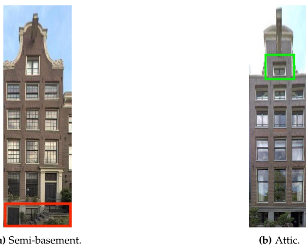
Figure 2.7.: The problem of which storey (types) to include in floor count is simplified to counting the total number of visible rows of windows and/or doors. We disregard the concepts of semi-basements or attics, as either are counted as a (full) storey.
