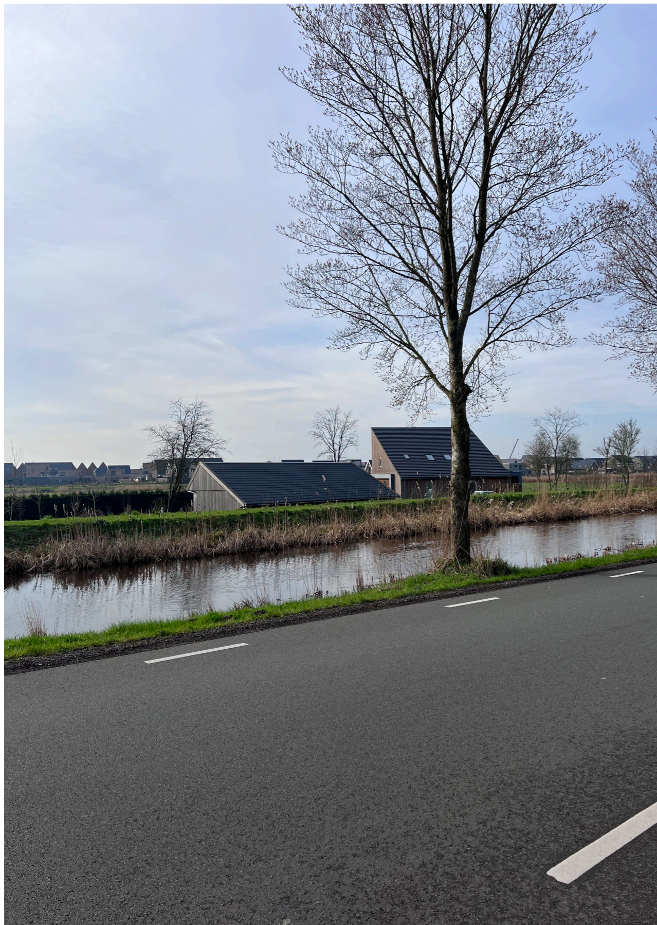
Figure 104 New buildings bellow the water level in Midden-Groningen, source: author
