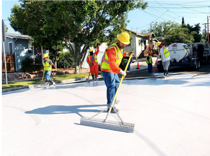
figure 7.24: Painting streets white in Los Angeles helped reduce the UHI effect (Abdallah, 2018).
