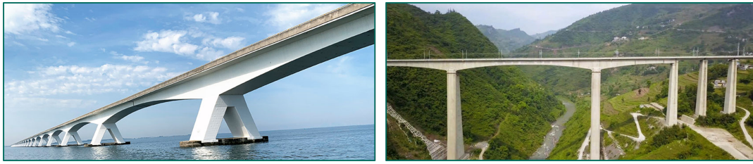
Figure 2.5: Concrete railway bridge examples with varying construction height. Specifically the Zeelandbrug and the Xiangbahe Railway Bridge
