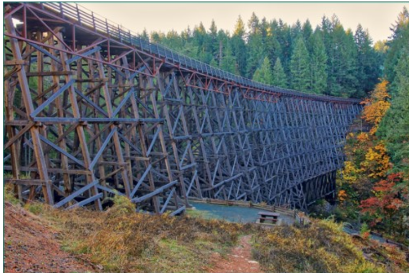
Figure 2.9: An example of a trestle bridge, the Kinsol trestle in Victoria, Canada.
