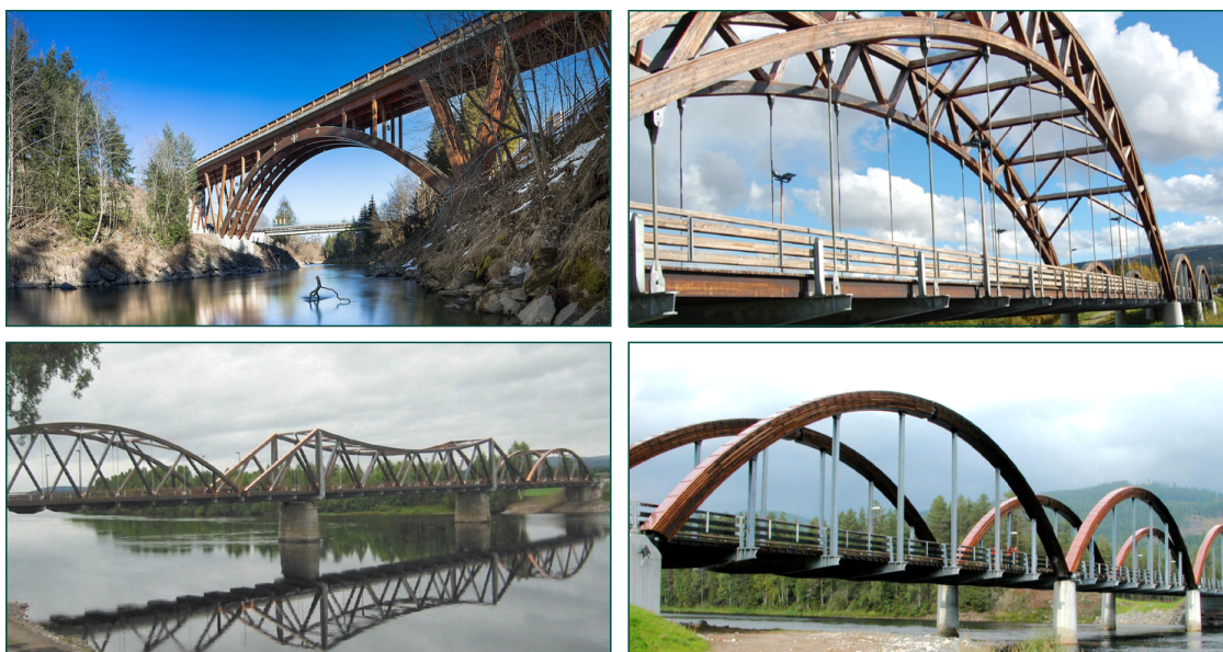
Figure 1.1: Examples of timber bridges. Wennerbrücke has a 45 metre span (top left), Tynnset bridge has a 70 metre span (top right), Flisa bridge also reaches 70 metre (bottom left), and Nybergsundbridge spans 40 metre (bottom right) (top left picture is of Pierer (2014), the other three of Aasheim (2019)).
