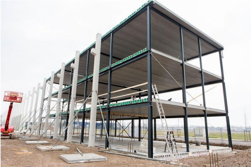
Figure 2.11: Example of concrete hollow core floors in building
