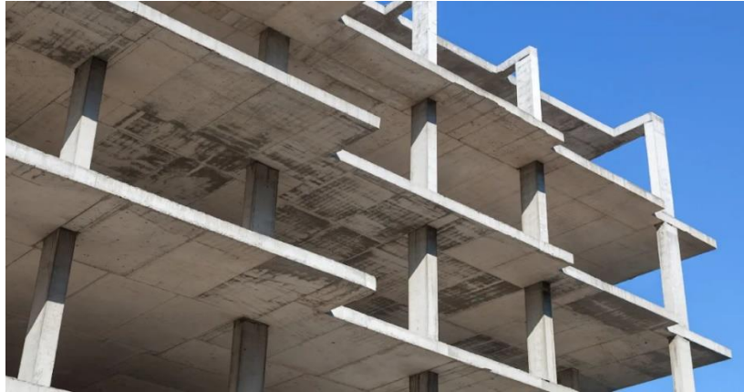
Figure 2.9: Example of a concrete cast insitu building
