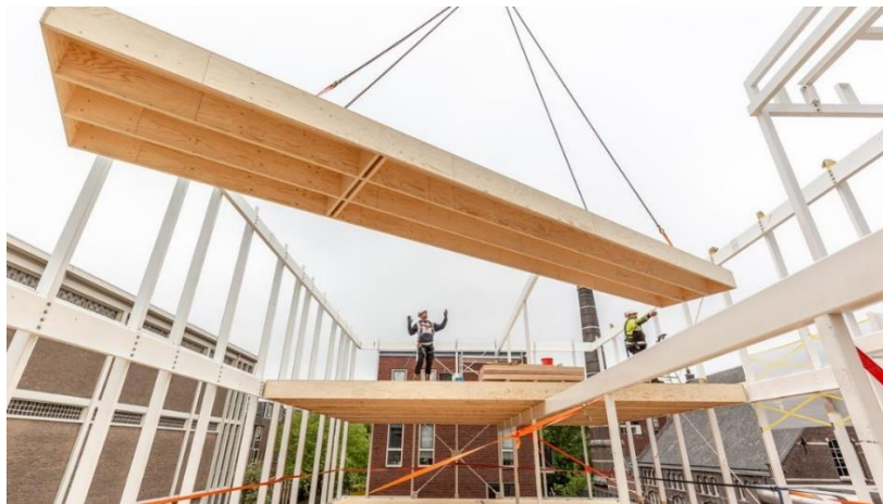
Figure 2.5: Example of a LVL floors (open box)
