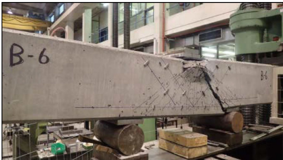
FIGURE 13 Beam B-6 after shear failure
