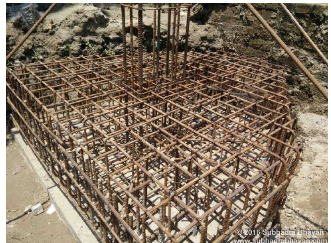
FIGURE 2 Reinforcement in a pile cap in traditional reinforced concrete
