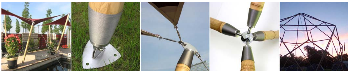
Figure 13: The jointing technique of the CONBAM building system developed by Christoph Toenges (CONBAM 2006).
