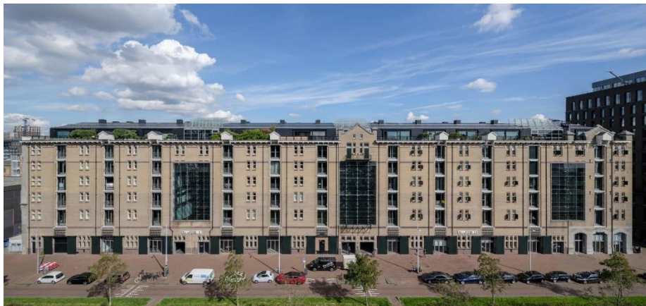
Figure 2.5 – St. Jobsveem Amsterdam
