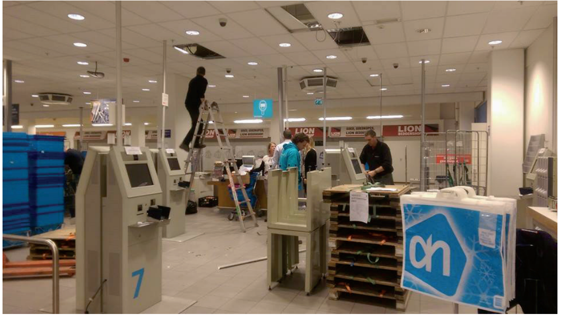
Figure 3.6 Decommissioning old supermarket lighting
