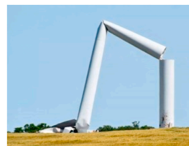
(c) support structure (tower) [27]
