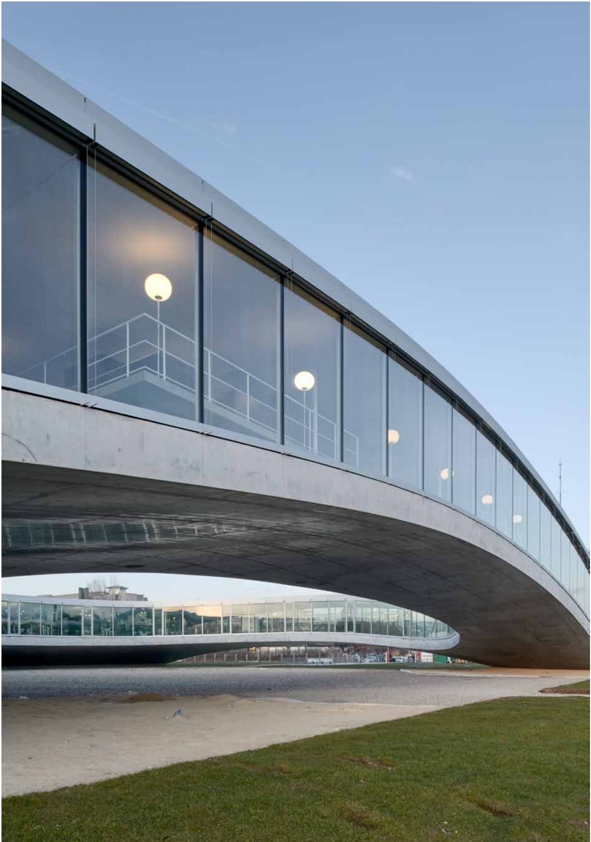
FIG. 5.5.1.7 View from South into large opening under VIP restaurant (Photo Ariel Huber)
