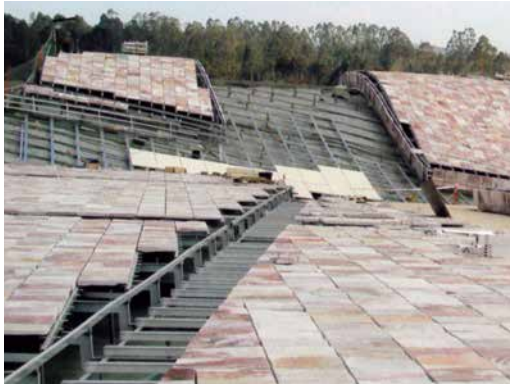
FIG. 6.4.1 Roof of newspaper archive under construction
