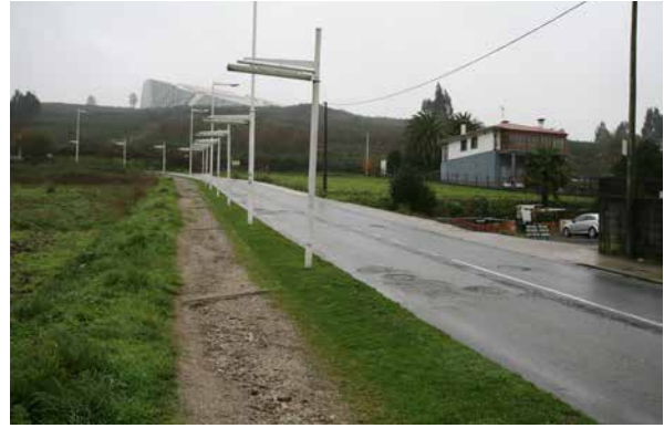
FIG. 6.3.2 ... a worksite abandoned after parliament ...
