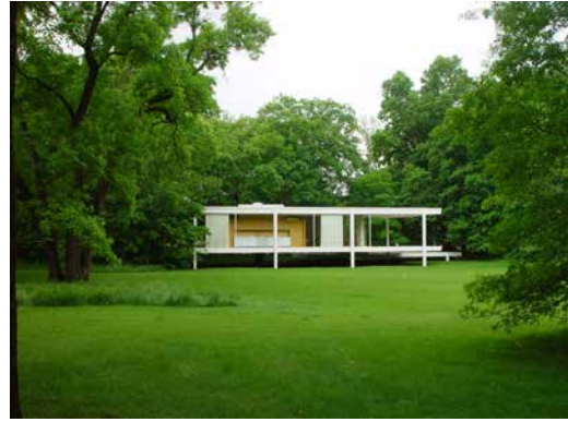
FIG. 3.1.8.2 Farnsworth House in Fox River floodplain
