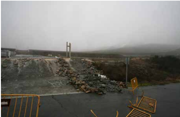
FIG. 6.3.3 ... decided to stop the unfinished project...
