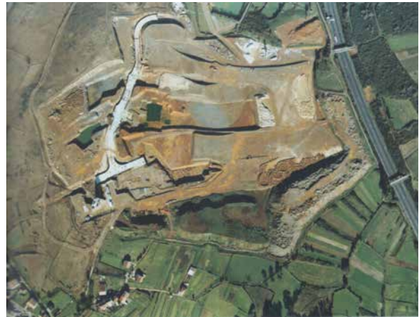
FIG. 6.5.1.13 Excavation w/ tunnel roof in 2003 (arqufuture 2009 p.45)
