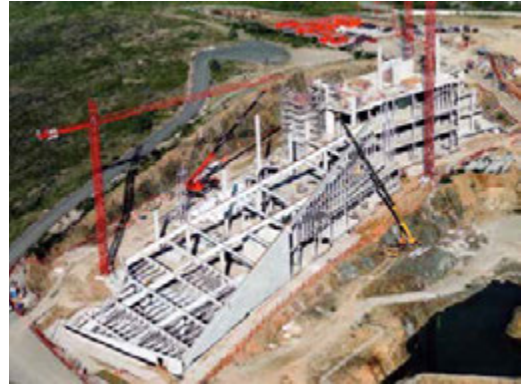
FIG. 6.4.2 central services under construction
