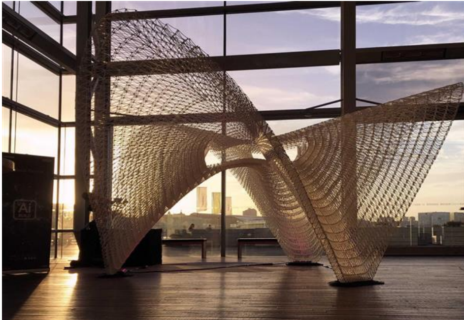
Figure 11: 3D printed Daedalus Pavilion at the GPU
