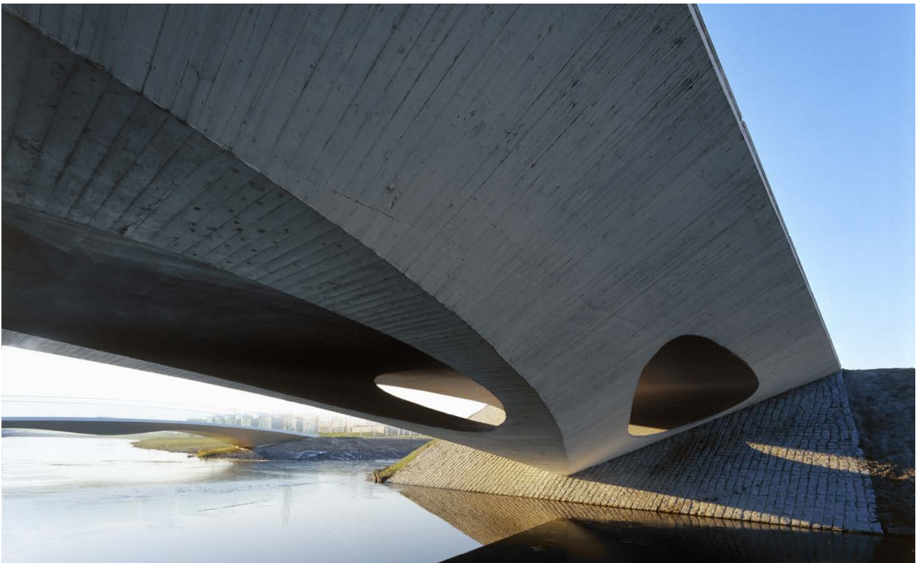
Figure 6: View on the intersecting cavities in the abutment on the water side. Clearly visible are the rough timber planks in the formwork of the vault and the sides. The cavities on the other hand are smooth inside
