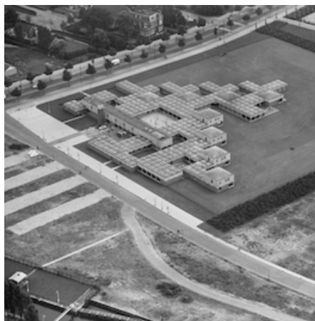
fig 4: Birds-eye view of the building in its (lack of) context
