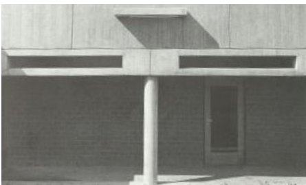
fig 24: The recurring structural elements of the building.
