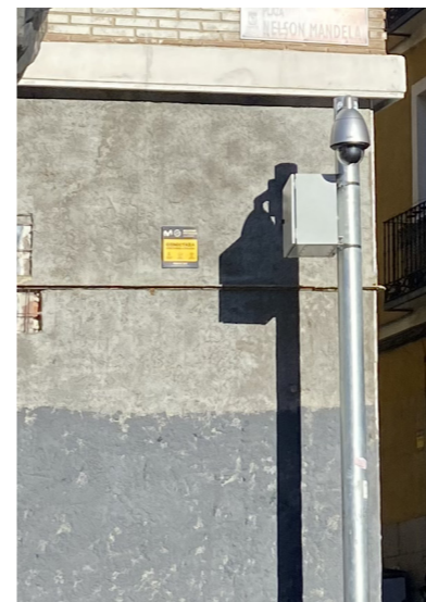
Camera on site visit (2023)
