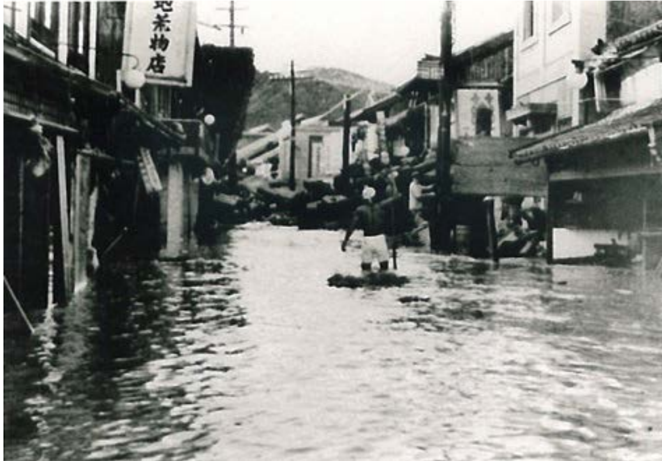
Flooding situation Yagi Town Typhoon No. 13, 1953
