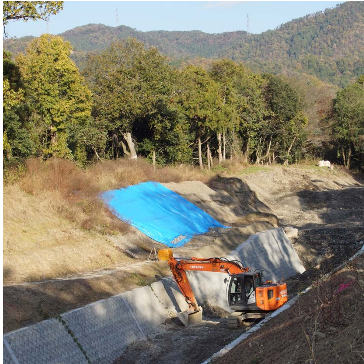
Nanatani River banks-soft edges are transformed into concrete hard edges.
