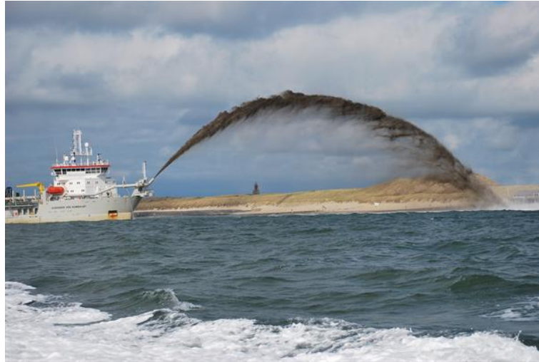
Figure 2.2. Sand nourishments in the Netherlands (Rijkswaterstaat, 2009)
