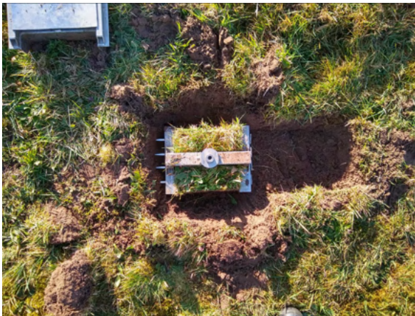
(c) Installing pull frame
