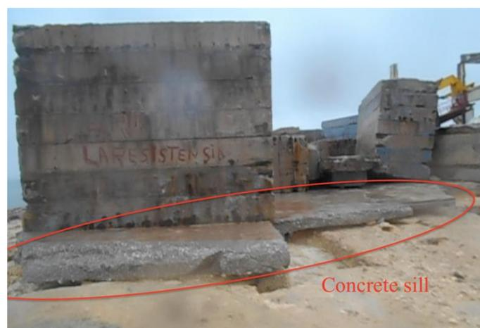
Figure 26 - Concrete sill as foundation for the old sea defense (Video footage of Hurricane Irma, 2017)
