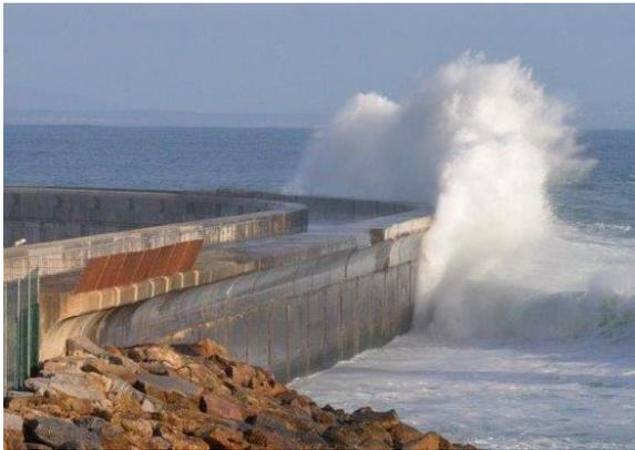
Figure 110 – Effective bullnose at Cascais, Portugal (Allsop, et al., 2018)
