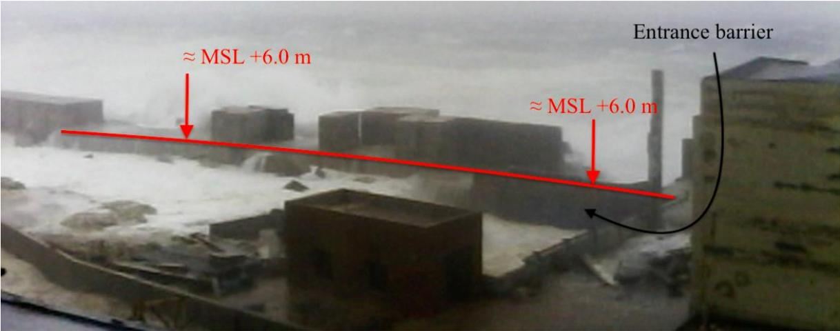
Figure 24 - height of the sill of the original barrier foundation
