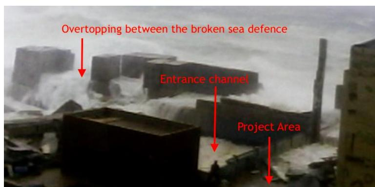
Figure 22 - Overview of entrance channel and overflow through broken sea defense (Video footage of Irma razing over the power plant, 2017)
