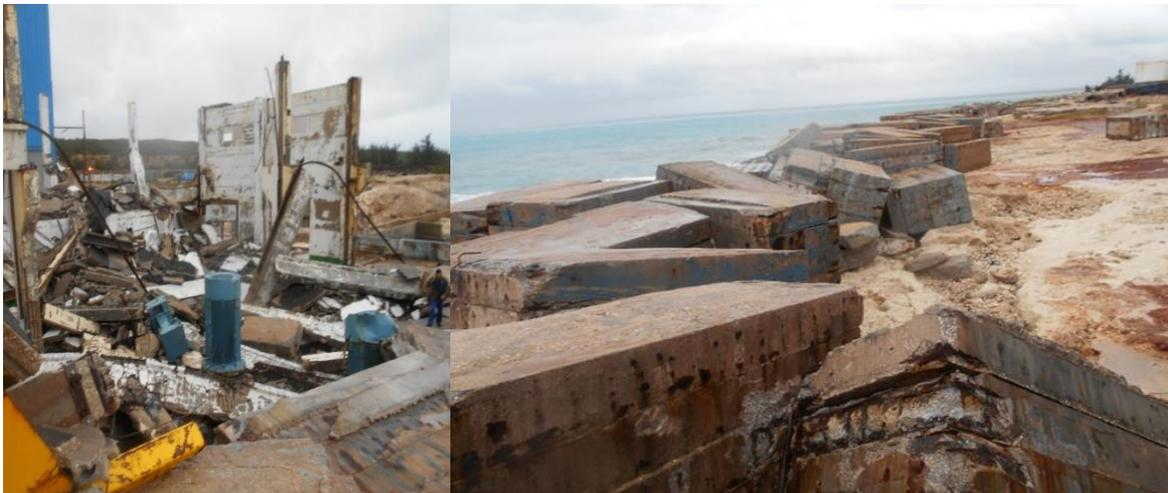
*Figure 4 - Damage of the thermoelectric power plant caused by hurricane Irma (Rubio Sauvalle, et al., 2018)*
