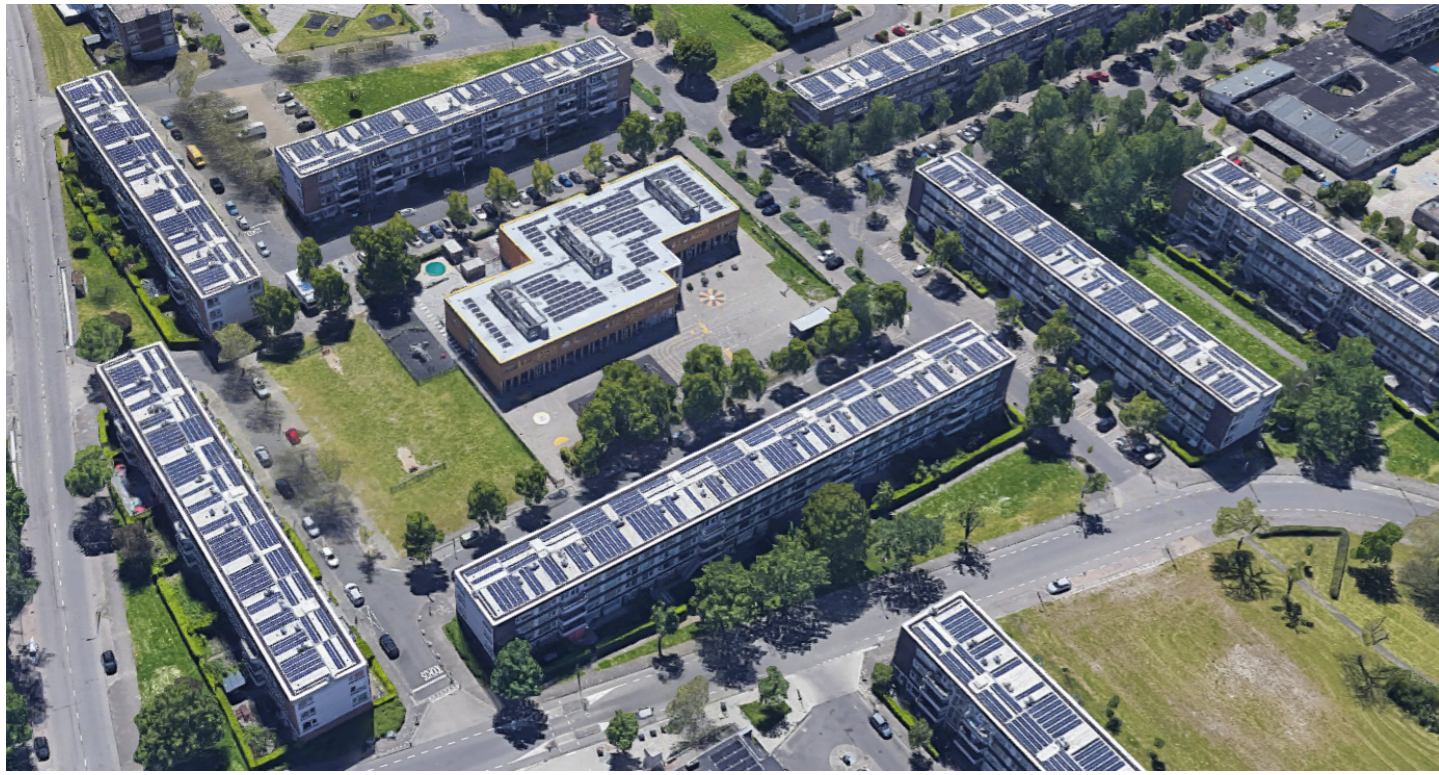
Figure 1.28. An example of the space in between the porch flats. The changes that have been made are mainly schools, which changes the view out of the dwellings onto the public space.
