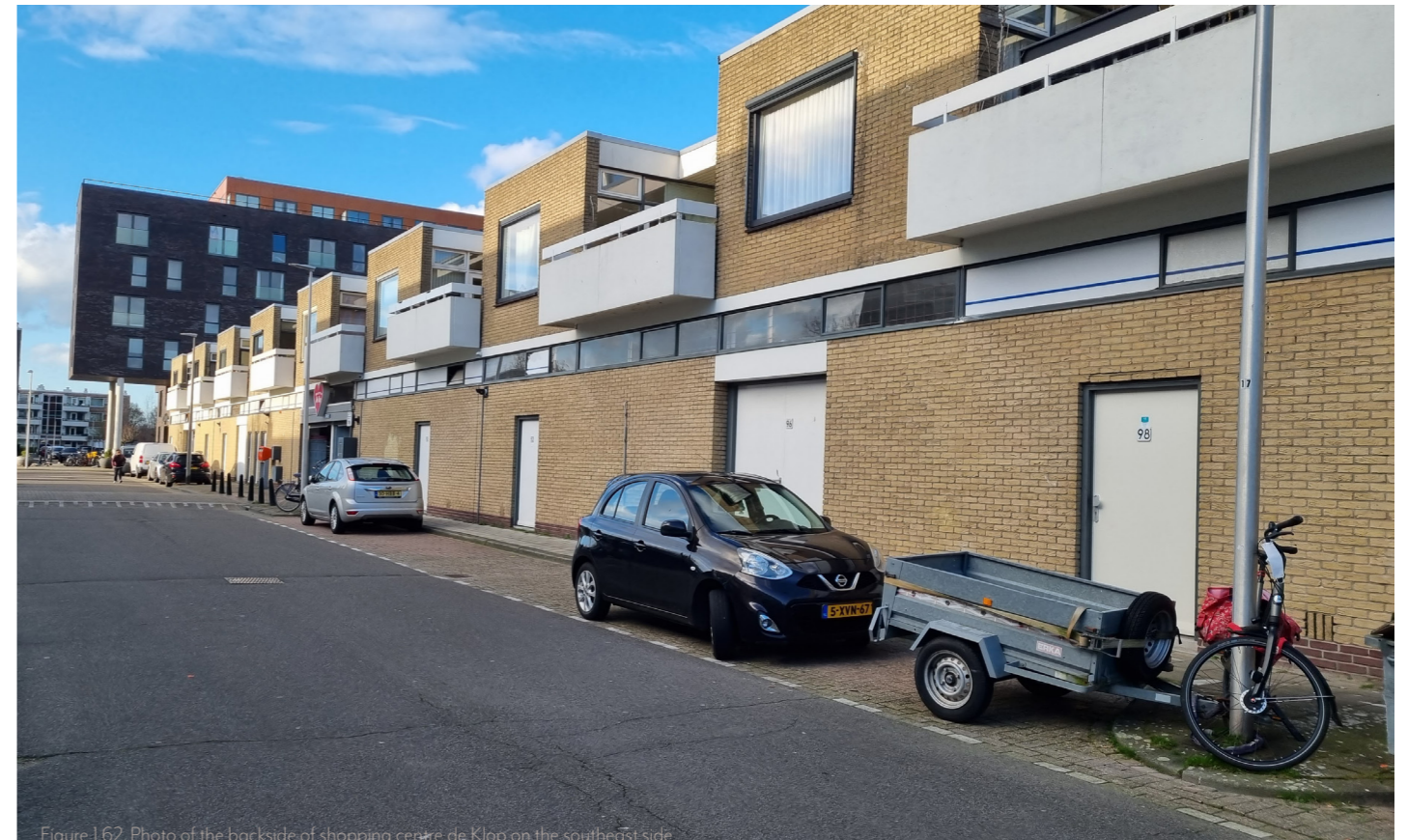
Figure 1.62. Photo of the backside of shopping centre de Klop on the southeast side
