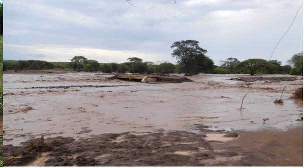
Figure 2.5: Broken bridge at C103 road, nearby Kuku
