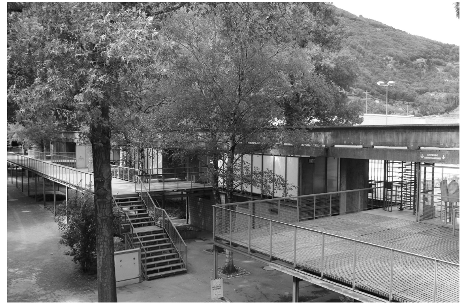
Access Platforms and Pathway, 2009
