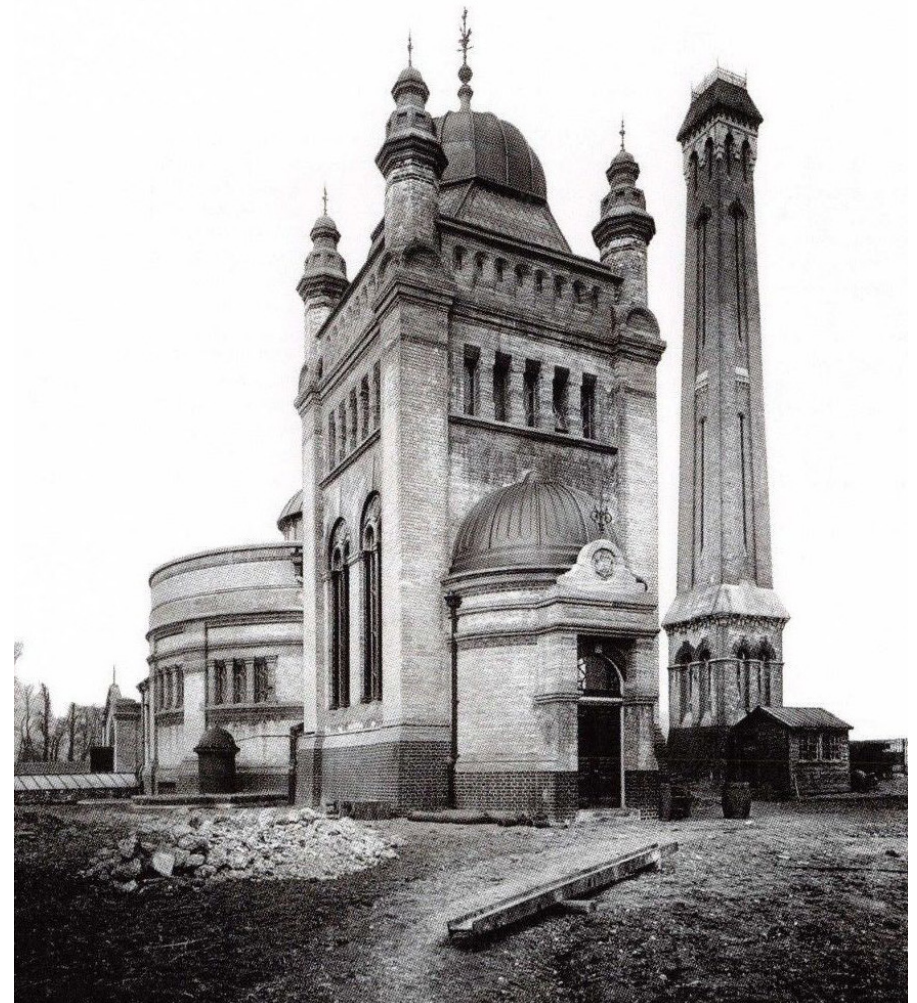
Streattham Pumping Station, 1895
