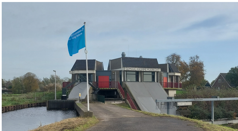
Figure 3.21: Pumping station with textile cover (Image courtesy of Witteveen+Bos)
