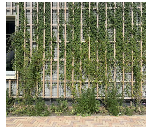
Wooden frame with steel wire and Clematis Vitalba.
