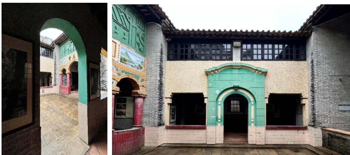
(Left) Figure 22. The rooms on the ground floor open directly to the outside.
