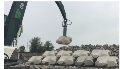
Figure 1.3: XblocPlus placement [16]
