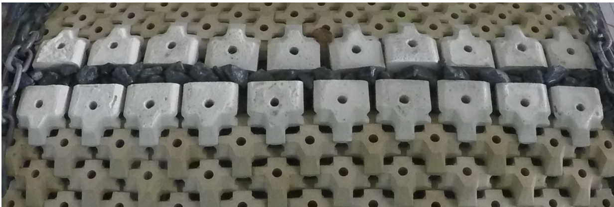
Figure 7.16: Crest armoured with starting blocks
