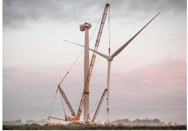
Figure 10.3 Siemens SWT-6.0-154, 120 m hub height,
