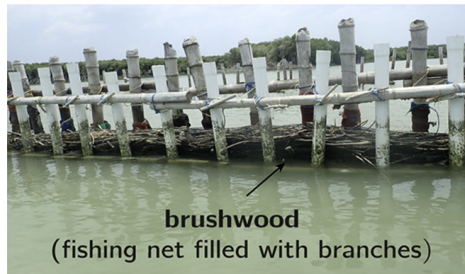
Figure 2.8: Permeable dam in use in the Indonesian coastal region. The vertical poles act as the framework supporting the brushwood bundles (picture courtesy of A. Gijón Mancheño)
