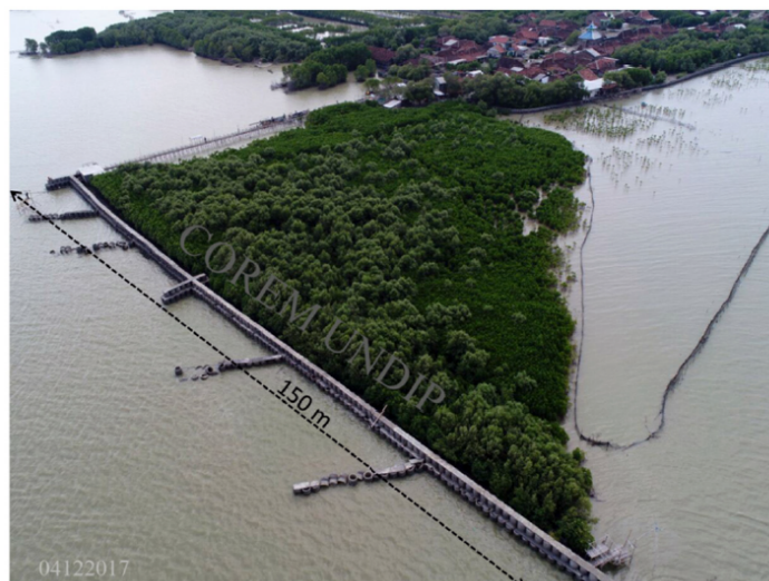
Figure 2.12: Seawall of concrete cylinders in Timbulsloko with the growth of dense mangrove forest behind the structure (picture courtesy of COREM-UNDIP)
