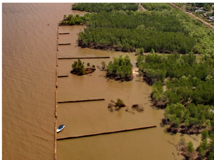
Figure 2.11: Wave damping observed behind the T-shaped dams in Vietnam (picture courtesy of R. Sorgenfrei).
