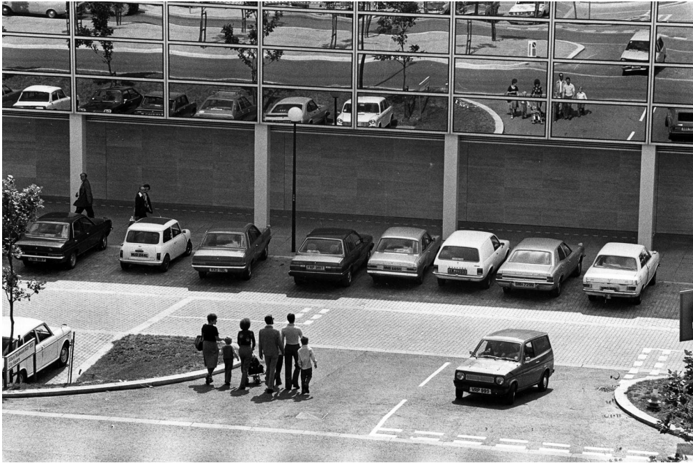
Figure 9. Exterior view of Milton Keynes' shopping centre, showing the mirror glass panels applied to the façade.
