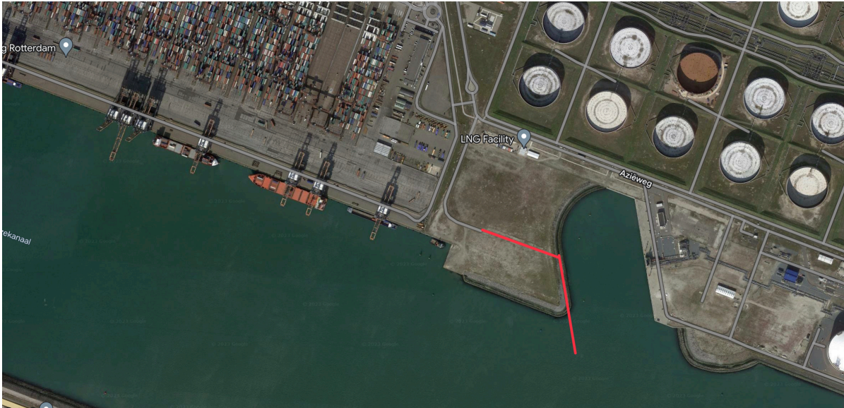
Figure 4.13: AAGV water/land transfer location at Euromax terminal, [41]
