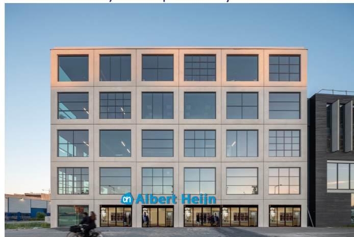
D1. Facade with large storefront (added for survey comparison)
