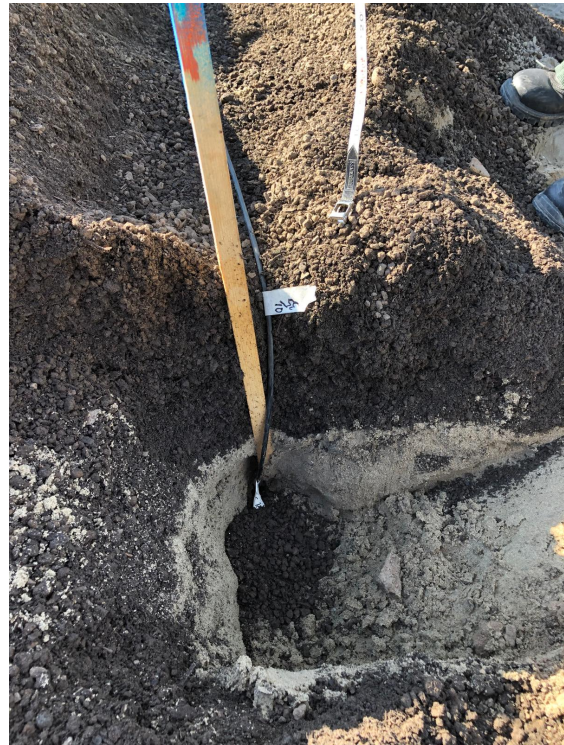
(b) Fibre-optic cable transitioning from deep to shallow section.
