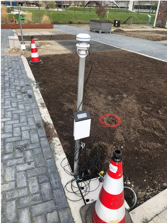
(a) Sensor hubs to which anemometers and tensiometers are connected.
