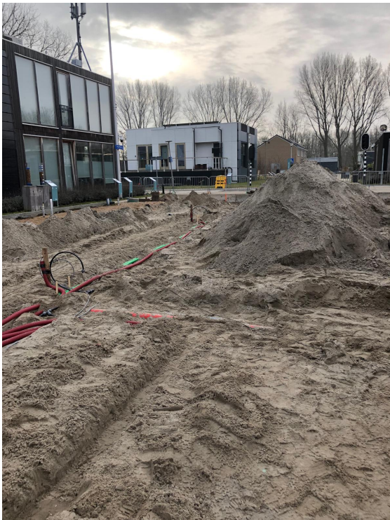
(a) Trenches dug at the required depth for the fibre-optic cable.
