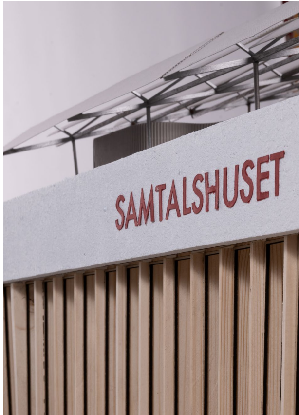
Close up of the facade.
