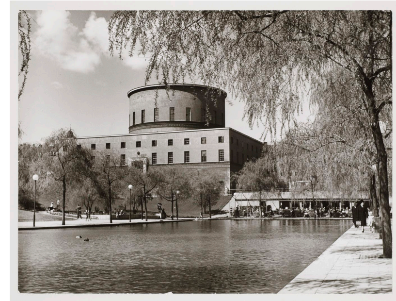
Archival photograph of the Asplundhuset.
