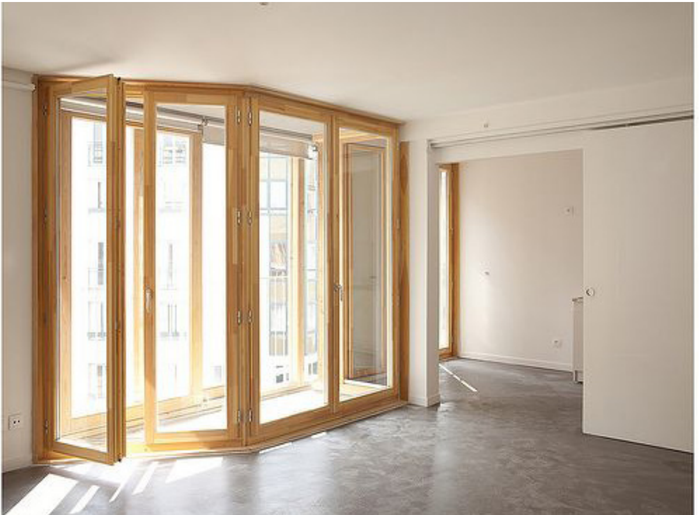
Top_ model of corner of the building, Antony Vajou Bottom_ Bioclimatic skin at its widest point; 1,50 m
