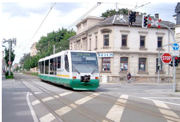
Figure 4-4: Train-tram on the Zwickau tram network. Also note the dual gauge.
