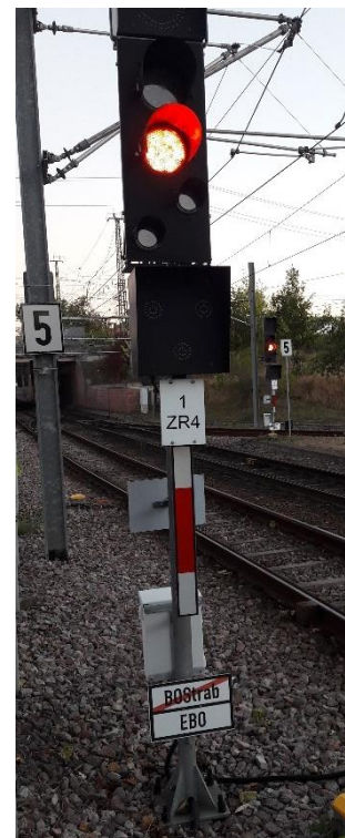
Figure 4-1: Start of EBO section. Note the small sign at the bottom.
