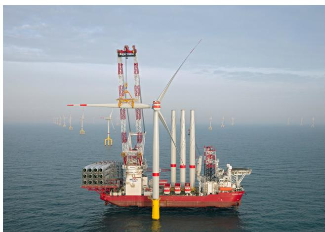
Figure 1.1: Jack-up installing an offshore wind turbine (Offshorewind, 2017)
