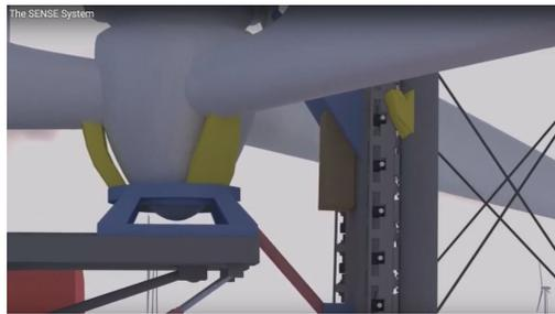
(a) Sense lifting method from vessel to carriage (Sensewind, 2017)
