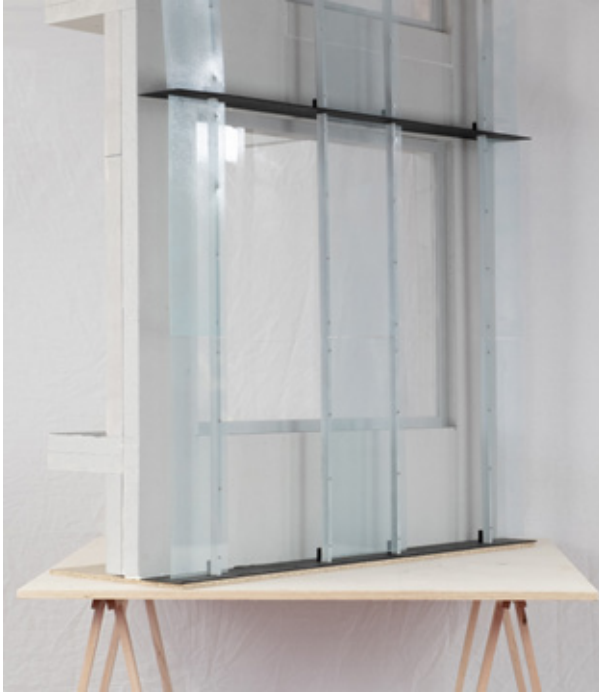
Fig. 11.7 Foam and polyester model of a fragment of the facade by Robbrecht and Daem, scale 1:5, Mees Wijnants and Tommaso Tellarini. Photograph: Bas Leemans.
