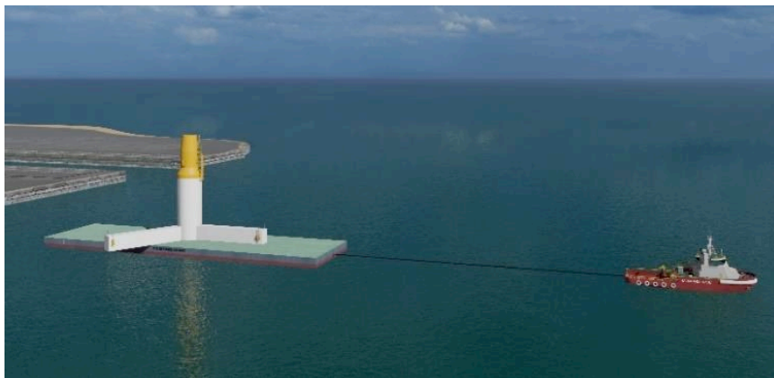
Figure 2-11 Float-out TLP floater (van der Nat, 2020)
