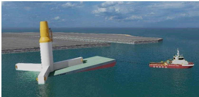
Figure 2-13 Load-out of TLP from barge (van der Nat, 2020)
